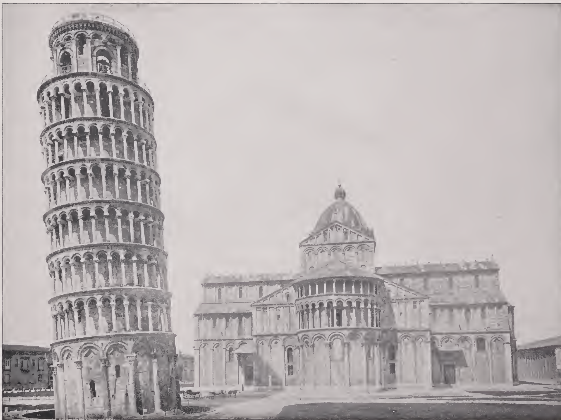
LEANING TOWER, PISA, ITALY —Pisa is principally noted for its famous "Leaning Tower," begun in 1174, and built of white marble; it is one hundred and seventy-eight feet high, and fronted with two hundred and seven columns. It is fifty feet in diameter, and leans thirteen feet from the perpendicular. The foundation being made insufficiently solid, it began to incline before it was one-third completed. The Cathedral on the right was begun in 1604, and consecrated in 1618 by Pope Gelasius; it contains the famous chandelier which Galileo saw swinging, and which led to his invention of the pendulum of the clock. The Baptistry, close by is noted for its marvelous echo.
